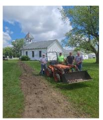
3. **Bonus Work -- Electricity:** The electricity to the garage and barn was routed from the house and a flawed set-up. All new underground electric from the church to the garage and barn for a safer and more efficient system has been installed. In addition, all power was discontinued from the house eliminating the second monthly electric bill. This work was done by church members and friends.
